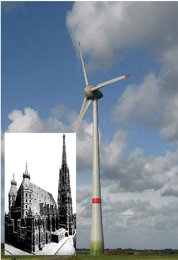
Enercon E-126: 7.5 MW, height 198 m, diameter of rotors 126 m
